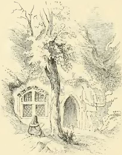
EXTERIOR VIEW OF ST. ROBERT'S CHAPEL, KNARESBOROUGH.
